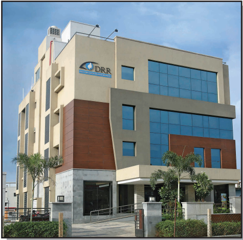
DRR Hospital No.399, Trunk Road, Karayanchavadi, Poonamalle, Chennai
